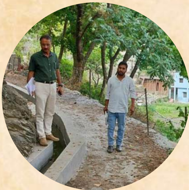
Irrigation Canal construction in Mulyagaon
