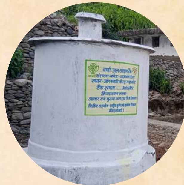
Rain Water Harvesting cum Storage Tank in Bidakot
