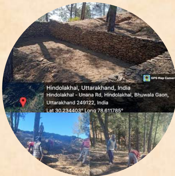
Percolation Tanks in Langur
