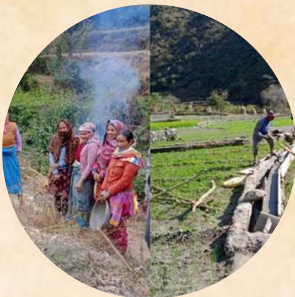
Repair of Irrigation Canal - Gadakot
