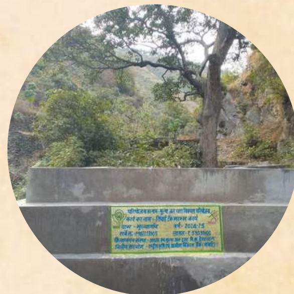
Repair of Irrigation Tank - Mulyagaon
