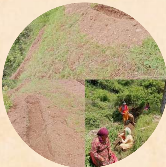
Staggered Contour Trenches - Langoor, Pansada
